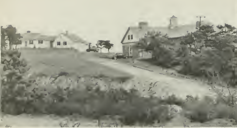
New transmitter building (right) and cottage occupied by engineer-in-charge.
